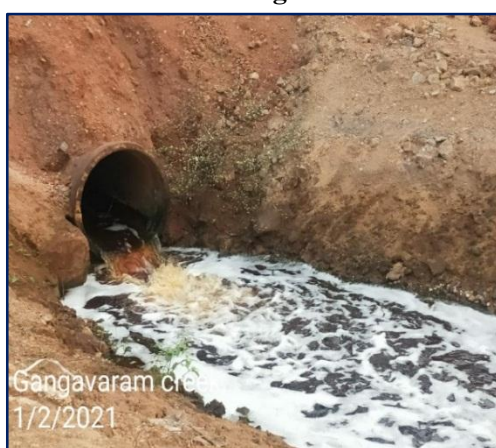
Discharge of untreated effluents into Gangavaram Creek
